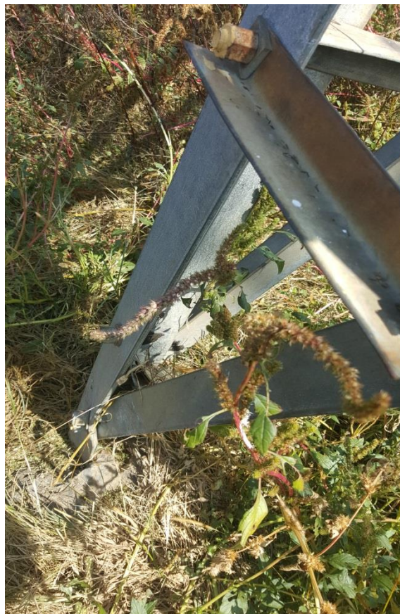
Figure 1.2: Damaged tower members on leg B
