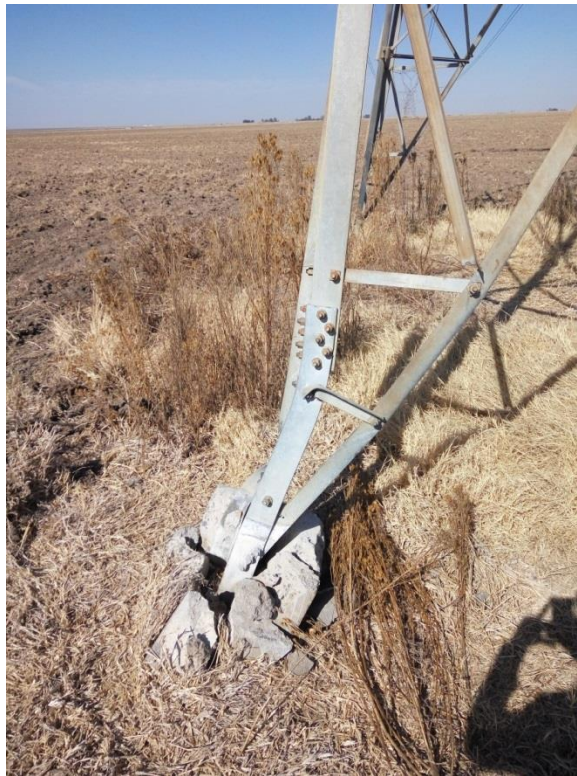
Figure 1.1: Damaged tower members on leg A
